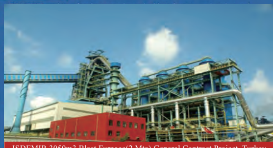
ISDEMIR 3050m3 Blast Furnace(2 Mta) General Contract Project, Turkey
