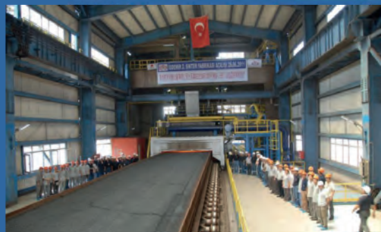
ISDEMIR 300m2 Sinter Plant, Turkey
