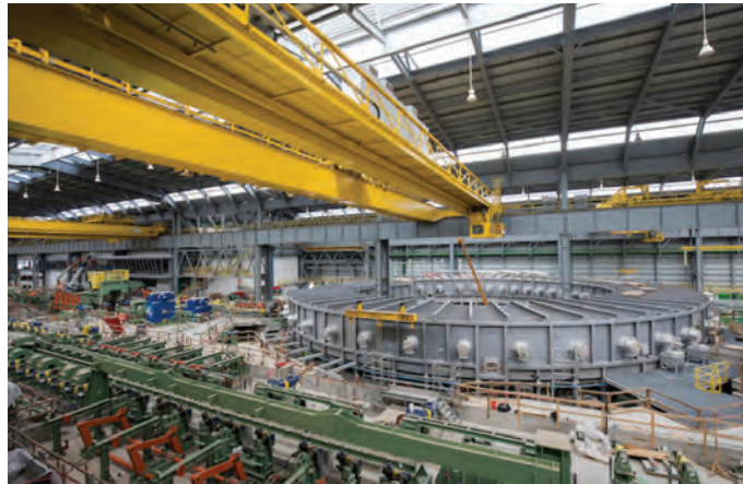
Tenaris' rotary furnace at Bay City, Texas
